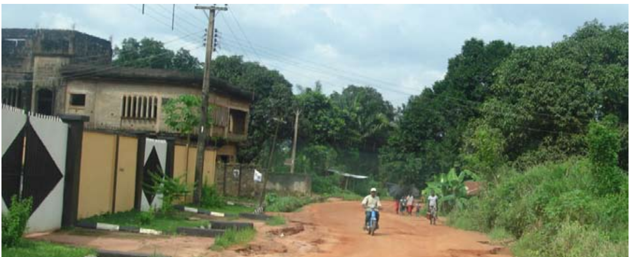
View of Erosion threat to residential areas.
